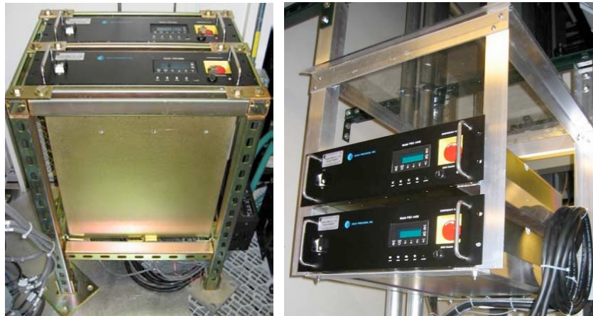
Figure 6. Custom made, single or dual-PSC mounts are space efficient and inexpensive
